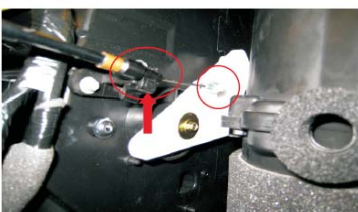
13 取掉空调拉线
